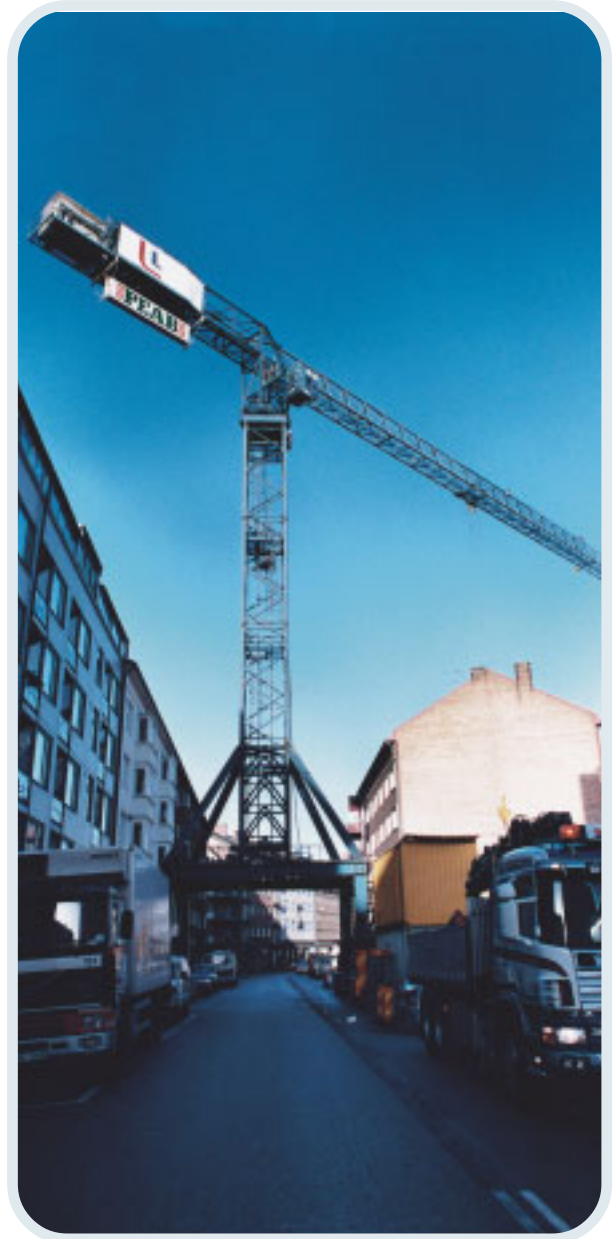
A crane from Lambertssons mounted on a gate over Engelbrekts-gatan in central Malmö wide enough for traffic in both directions
