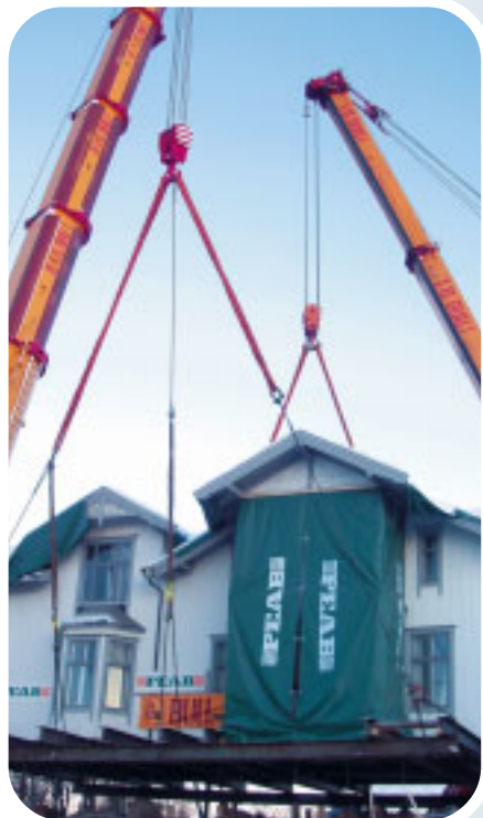
Moving house in conjunction with the expansion of Asker's Station in Oslo.
