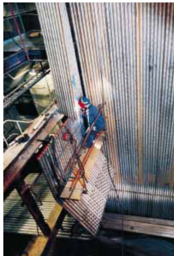
Sandvik's composite tubes withstand the aggressively corrosive environments in waste incineration plants.
