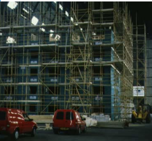
In a hangar in Cardington in Great Britain, a six-storey building is being constructed of timber. The intention is to carry out various tests and to demonstrate to European customers how such a building can be constructed.
