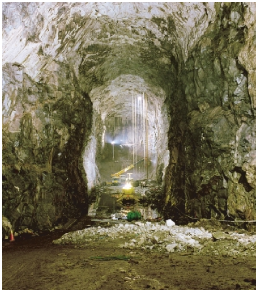
SYDKRAFT GAS CONVERTED A FORMER UNDERGROUND OIL STORAGE CHAMBER INTO A REFRIGERATED LPG STORAGE UNIT DURING 1999.
