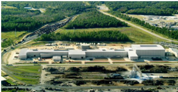
▲ The new quenching line in Mobile.
