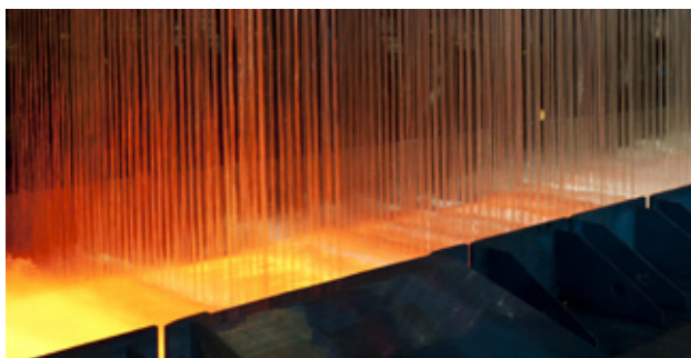
▲ The new quenching line in Borlänge.
